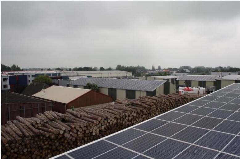
The local IBC SOLAR partner company Xperal was in charge of the installation. Altogether, there were 9,240 modules installed on the rooftops of Plospan, a wood processing company in Waardenburg. With this many modules, the system is now the biggest PV installation in the province of Gelderland.
