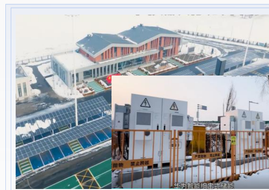
Qunli toll station @ northern china -30°C, severe cold
