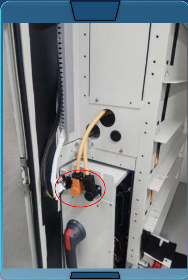
B+ and B- of tower
